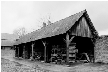
Hangar. Phot. Benoît Dufournier IVR22_19888000097Z
