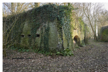
Aile ouest. Caponnière simple. Phot. Pierre Thibaut IVR32_20235900153NUCA
