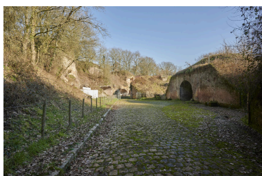
Cour ouest. Phot. Pierre Thibaut IVR32_20235900143NUCA
