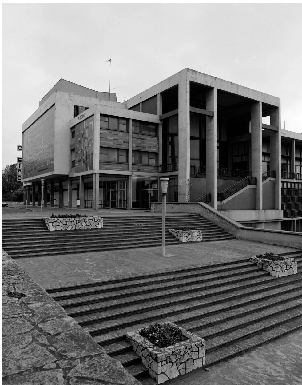
Casino municipal, angle nord.
