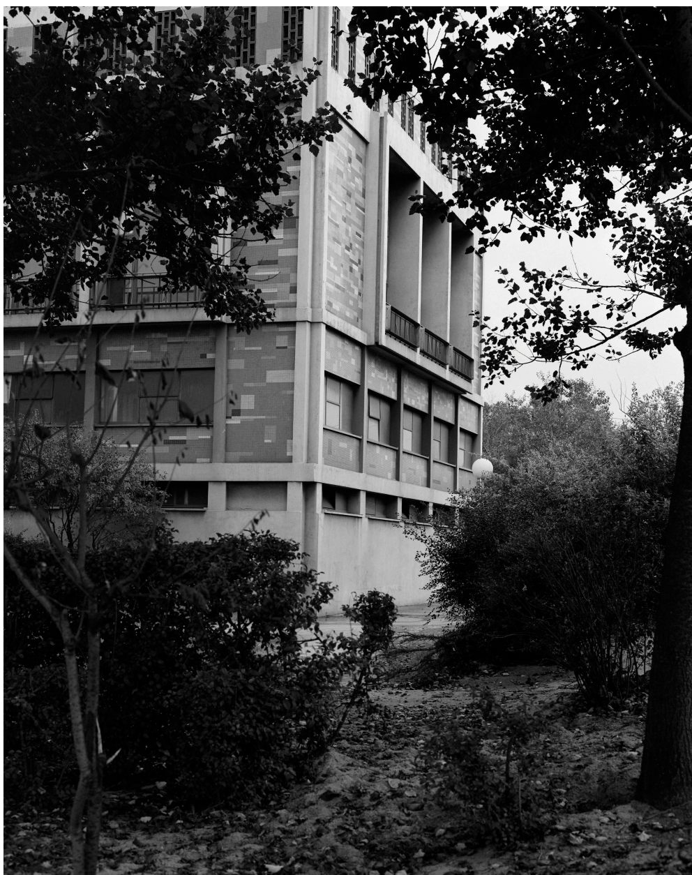
Casino municipal, pignon sud.
