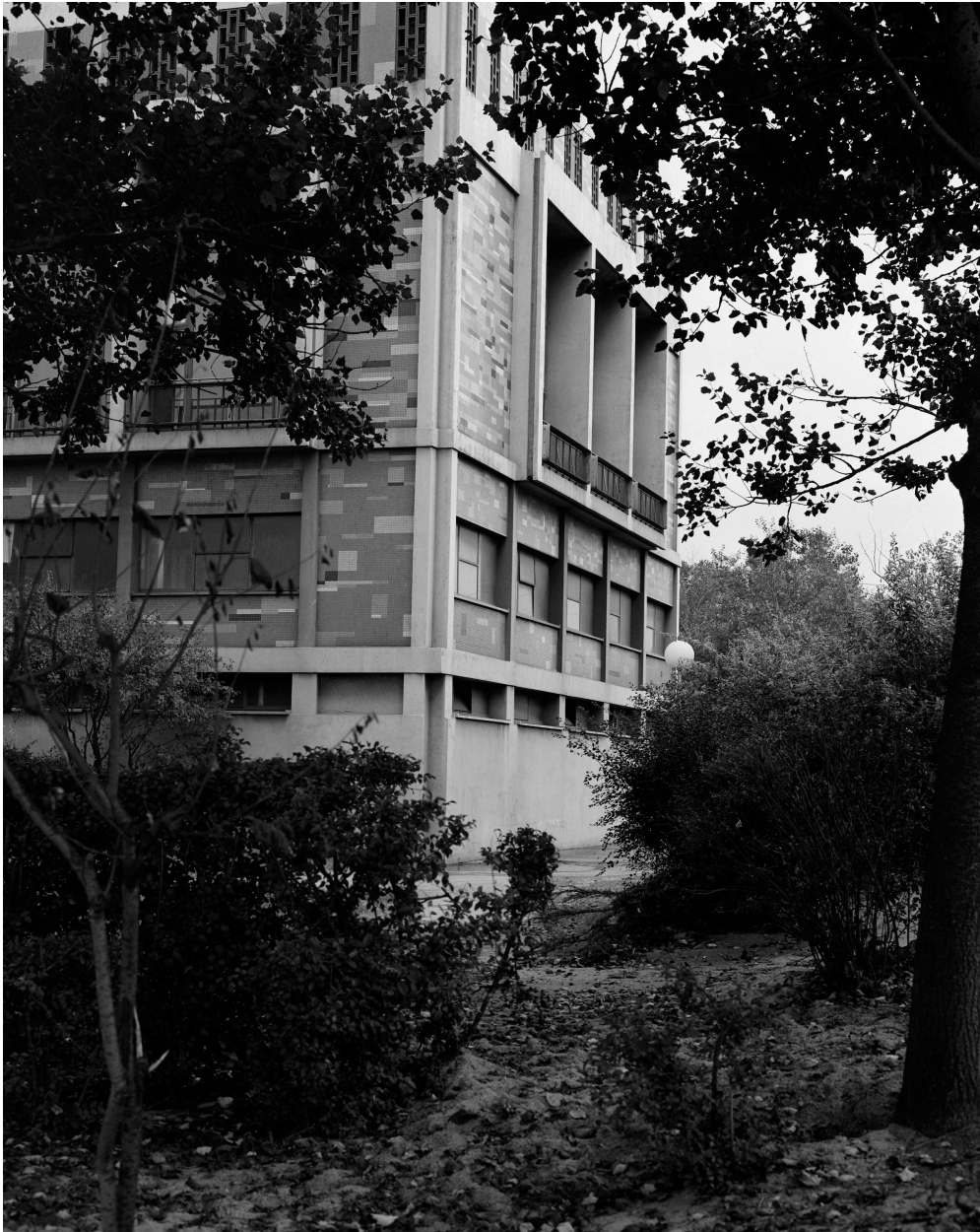
Casino municipal, pignon sud.
