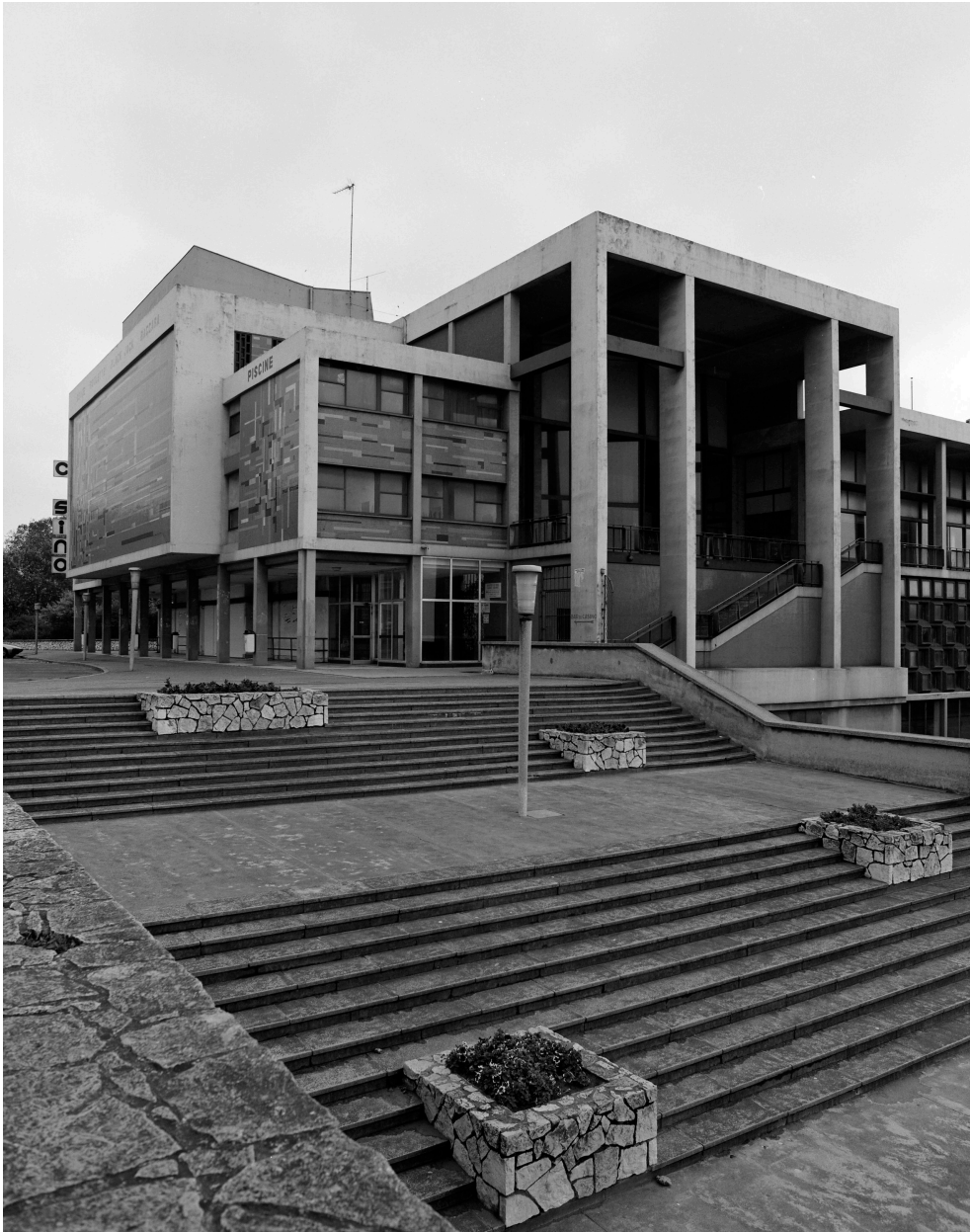
Casino municipal, angle nord.
