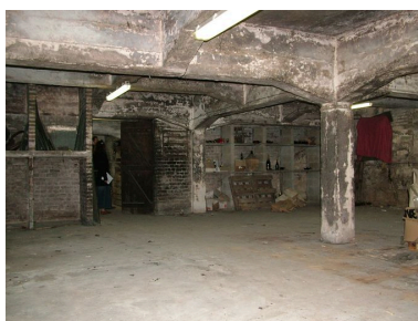
Vue des caves. Phot. Irwin Leullier IVR22_20050200958NUCA
