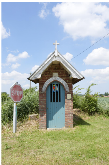
Face avant. Phot. Delphine Volto-Jourdan IVR32_20245902474NUCA
