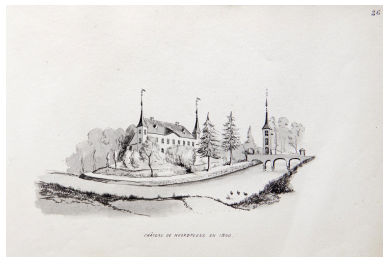
Château de la Tour, Noordpeene, gravure, 1860. In Album Flahaut XIXe siècle (Comité Flamand de France). Repro. Delphine Volto Jourdan IVR32_20255900782NUCA
