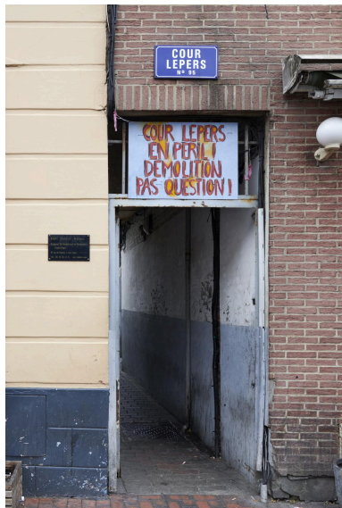
Entrée Cour Lepers. Phot. Delphine Volto Jourdan IVR32_20265900131NUCA
