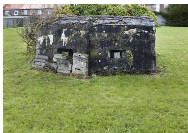
Elévation nord Phot. Jean-Marc Ramette IVR31_20145904292NUCA
