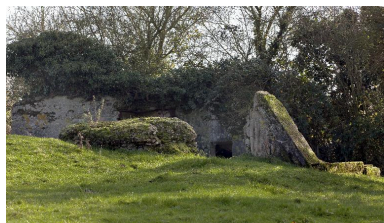
Elévation nord Phot. Jean-Marc Ramette IVR31_20145904882NUCA
