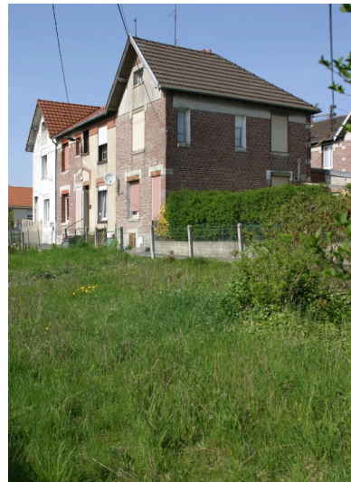
Pavillon de 1925. Phot. Frédéric Pillet IVR22_20070205159NUCA
