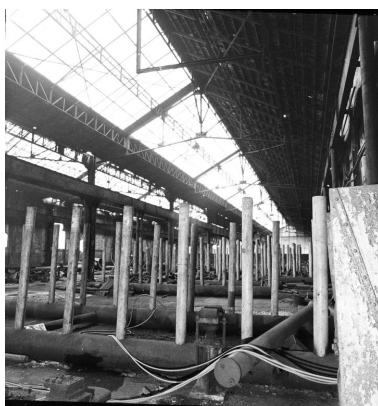
Aire de stockage des tubes (usine B). Phot. Olivier Marlard IVR31_19905900071X
