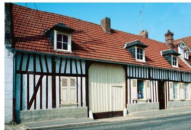
Elévation antérieure, de trois-quarts. Phot. Alain Nafilyan IVR22_19856001321ZA
