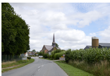
Entrée sud du village de Wemaers-Cappel. Phot. Delphine Volto-Jourdan IVR32_20235901221NUCA
