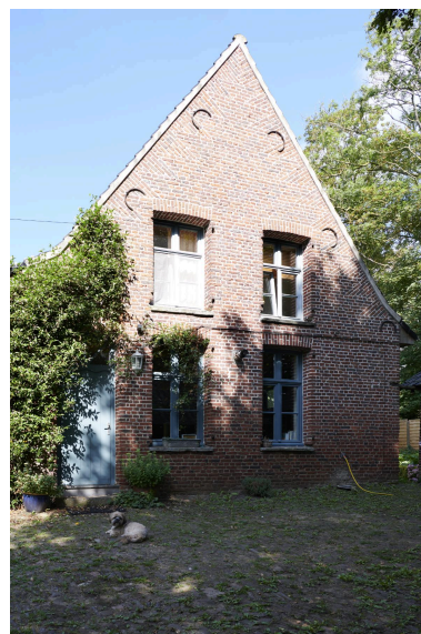
Pignon est. Phot. Delphine Volto Jourdan IVR32_20245902813NUCA
