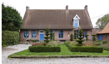
Logis de la ferme. Phot. Delphine Volto Jourdan IVR32_20255900441NUCA
