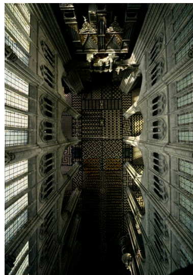
Dallage de la nef. Phot. Fabrice Charrondière IVR22_19868000040PA
