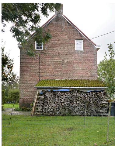
Pignon est. Phot. Delphine Volto Jourdan IVR32_20245903106NUCA
