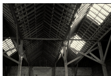
Charpente de la grange. Phot. Jean-Michel Perrin IVR22_19846001347X
