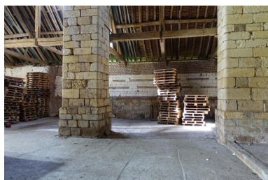
Piliers. Phot. Lucile Chamignon IVR32_20226005083NUCA
