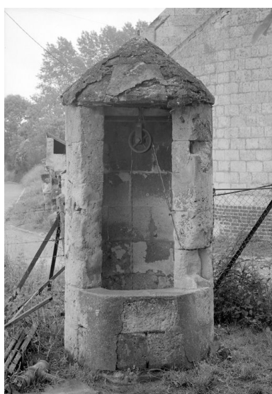
Puits. Phot. Jean-Michel Perrin IVR22_19856000777X
