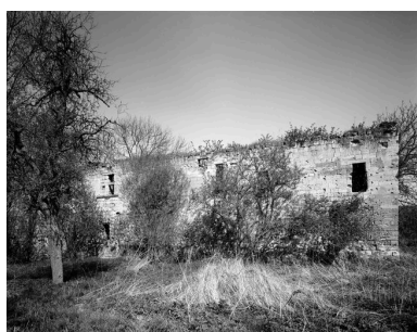
Elévation sud. Phot. Jean-Michel Perrin IVR22_19856000585V
