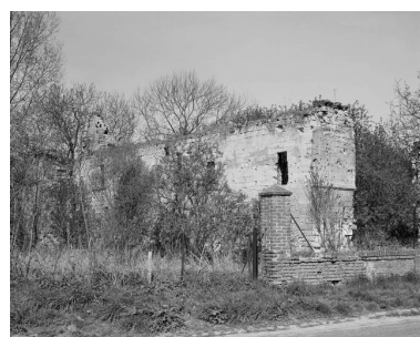
Elévation sud. Phot. Jean-Michel Perrin IVR22_19856000584V
