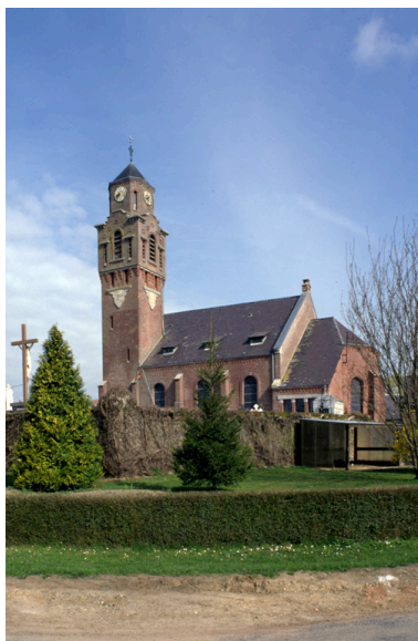
Elévation sud. Phot. Christiane Riboulleau IVR22_19960200462ZA
