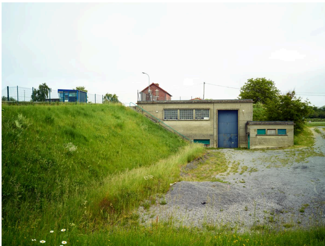
La station de pompage.
