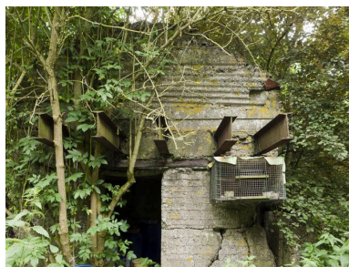
Elévation nord Phot. Jean-Marc Ramette IVR31_20145904427NUCA
