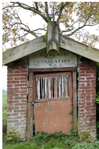
Façade principale. Phot. Delphine Volto Jourdan IVR32_20245902625NUCA
