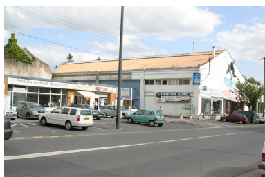
Atelier, boulevard Henri-Martin. Phot. Frédéric Pillet IVR22_20050206055NUCA
