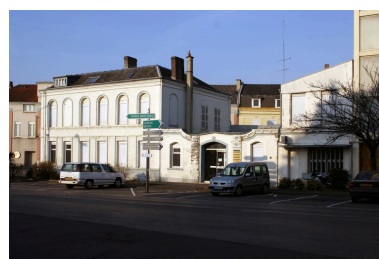
Façade antérieure, boulevard Gambetta. Phot. Frédéric Pillet IVR22_20050206177NUCA
