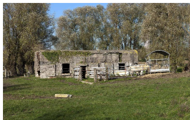
Elévation Sud Phot. Jean-Marc Ramette IVR31_20145904876NUCA
