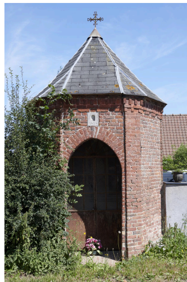
Façade principale. Phot. Delphine Volto Jourdan IVR32_20245902790NUCA
