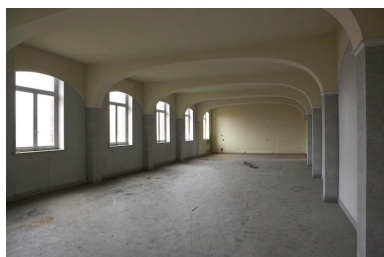
La chapelle. Phot. Pierre Thibaut IVR31_20095903356NUCA
