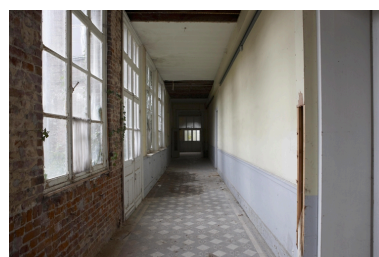
Le couloir reliant les ailes. Phot. Pierre Thibaut IVR31_20095903332NUCA
