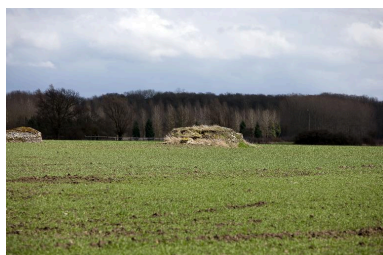
Casemate sud Phot. Jean-Marc Ramette IVR31_20146203036NUCA
