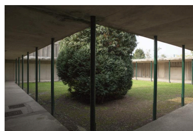
Cloître. Phot. Pierre Thibaut IVR31_20155900180NUCA
