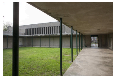
Cloître. Phot. Pierre Thibaut IVR31_20155900182NUCA
