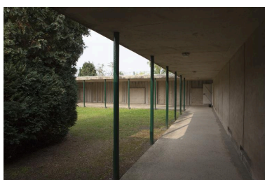
Cloître. Phot. Pierre Thibaut IVR31_20155900179NUCA
