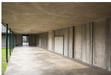
Cloître. Phot. Pierre Thibaut IVR31_20155900183NUCA
