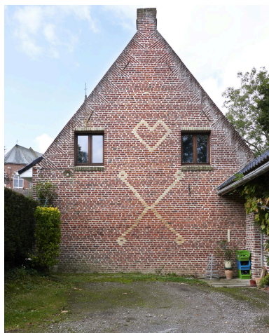
Pignon est. Phot. Delphine Volto Jourdan IVR32_20245903127NUCA
