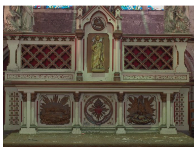
Vue partielle Phot. Bruno Decrock IVR31_20106201877NUCA
