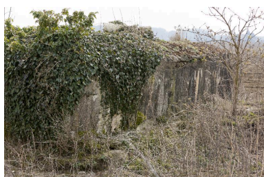
Elévation nord Phot. Jean-Marc Ramette IVR31_20145904007NUCA
