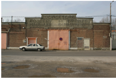
Atelier, quai Gayant. Phot. Frédéric Pillet IVR22_20050206196NUCA
