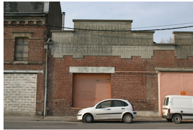
Atelier, quai Gayant. Phot. Frédéric Pillet IVR22_20050206197NUCA
