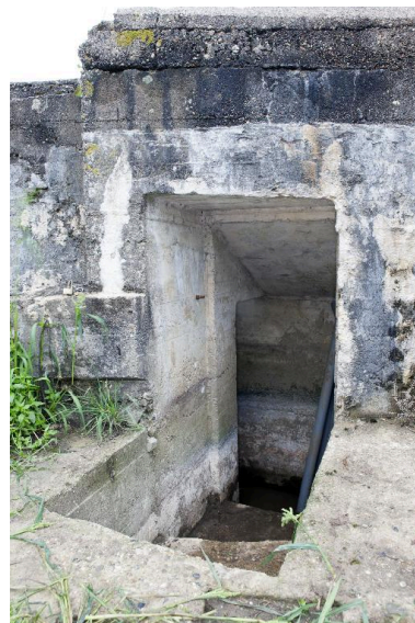
Entrée est. Phot. Pierre Thibaut IVR31_20155901484NUCA
