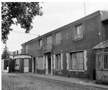
Logement patronal. Phot. Patrick Glotain IVR22_19936000742X
