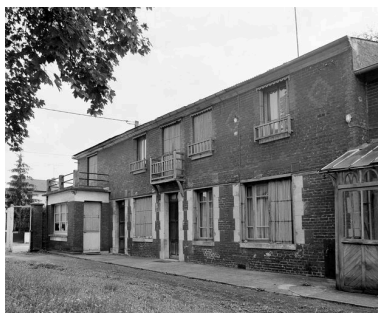
Logement patronal. Phot. Patrick Glotain IVR22_19936000742X
