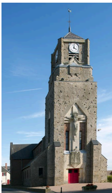
Façade principale est. Phot. Marie-Laure Monnehay-Vulliet IVR32_20188000601NUC2A
