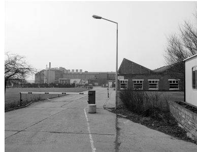
Bureaux, atelier de fabrication. Phot. Olivier Marlard IVR31_19915900098X
