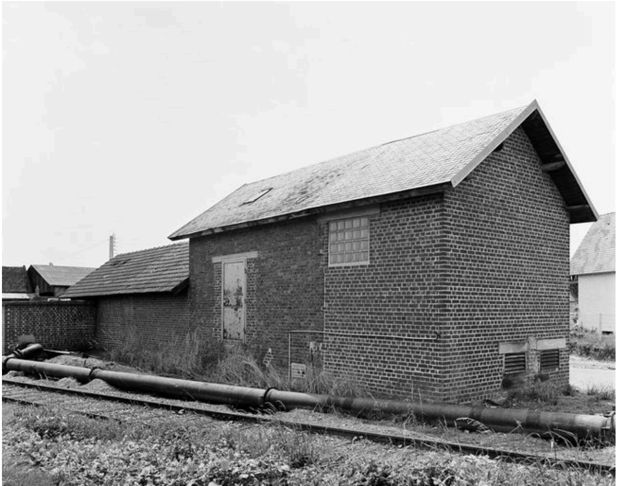
Station de pompage.
