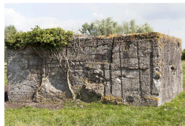
Elévation nord. Phot. Jean-Marc Ramette IVR31_20145905363NUCA
