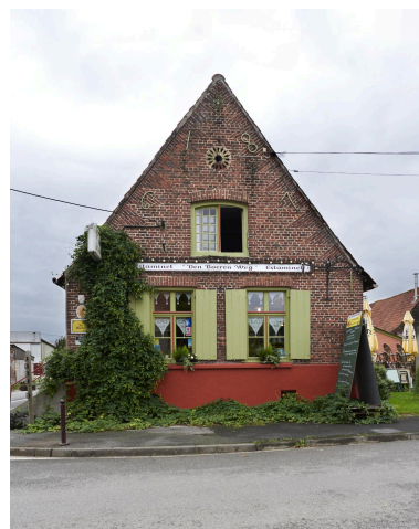
Pignon est. Phot. Delphine Volto Jourdan IVR32_20245902951NUCA
