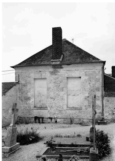
Pignon est. Phot. Jean-Michel Perrin IVR22_19846001061X
