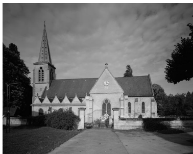
Elévation sud. Phot. Jean-Michel Perrin IVR22_19846001306V
