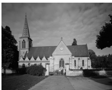
Elévation sud. Phot. Jean-Michel Perrin IVR22_19846001306V
