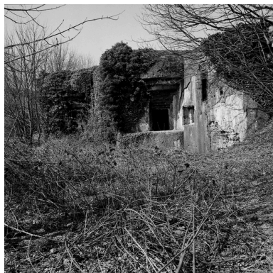
La casemate est. Phot. Philippe Dapvril IVR31_20045900202X
