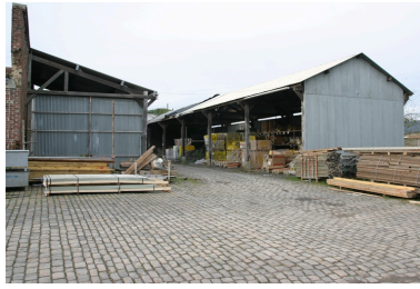
Hangars. Phot. Frédéric Pillet IVR22_20070205068NUCA
