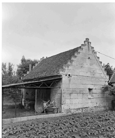
Remise. Phot. Benoît Dufournier IVR22_19946001334Z
